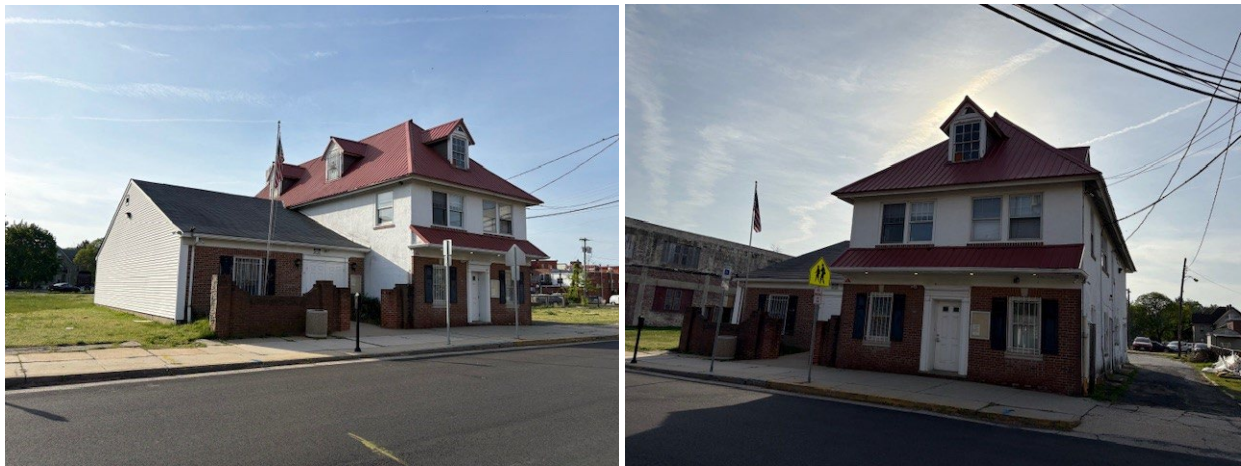
Photos: BRS site visit 29 April 2025
