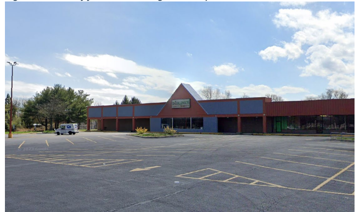
Figure 13: Site of former Incollingo’s Family-Owned Markets
