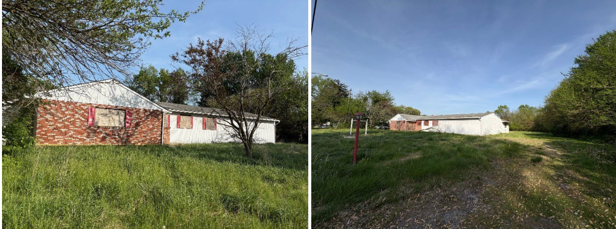
Photos: BRS site visit 29 April 2025
