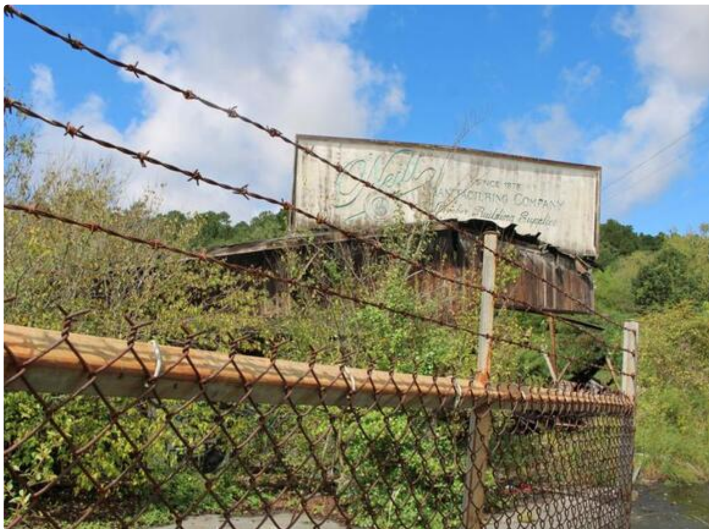
One of the county's most notable brownfield sites is the former O'Neill Manufacturing plant, a 7-acre tract off Anderson Street in North Rome. File, John Bailey
