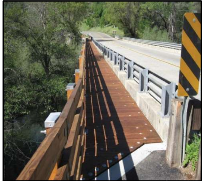
Above: Shared-use path cantilevered off an existing bridge. Source: Small Town and Rural Design Guide
