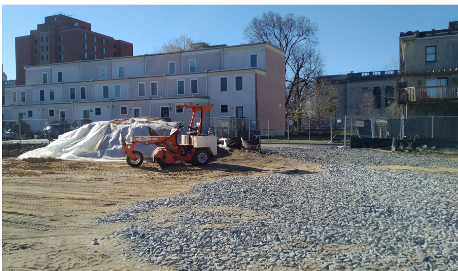
Site Remediation in Progress ABC Barrel Site, Camden, New Jersey
