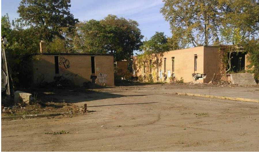
Camden Labs Existing Conditions
