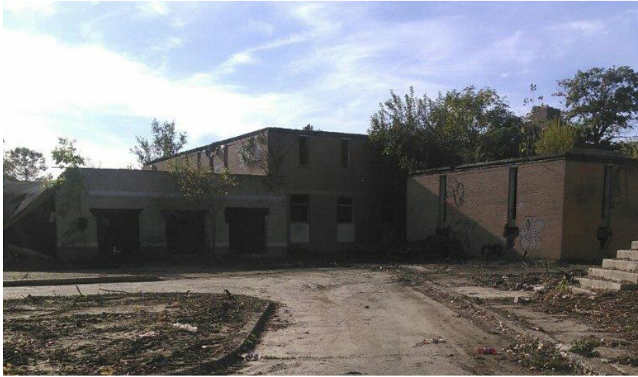
Catalyst Site - Camden Labs Prior to Assessment and Remediation, Fall 2016
