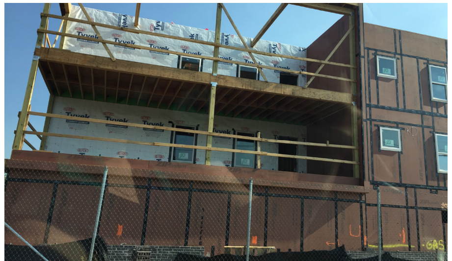
Centerville Neighborhood Branches at Centerville Housing Under Construction (Summer 2017)
